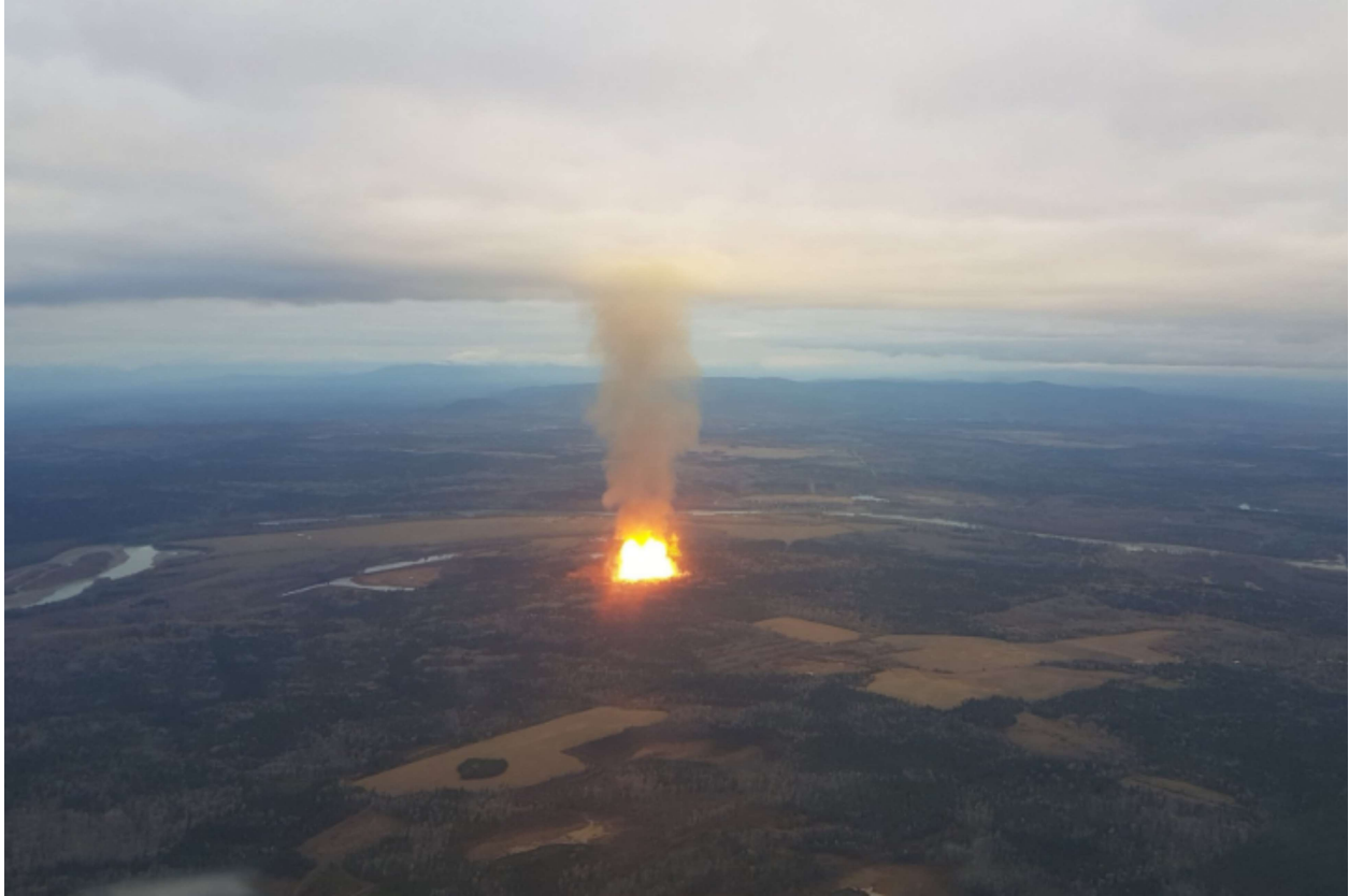
Figure 3.1.3 - Explosion at an Enbridge natural gas pipeline that impacted the Lheidli T'enneh First Nation in British Columbia, Canada ( https://globalnews.ca/news/4531677/prince-george-fire-evacuation/ )
