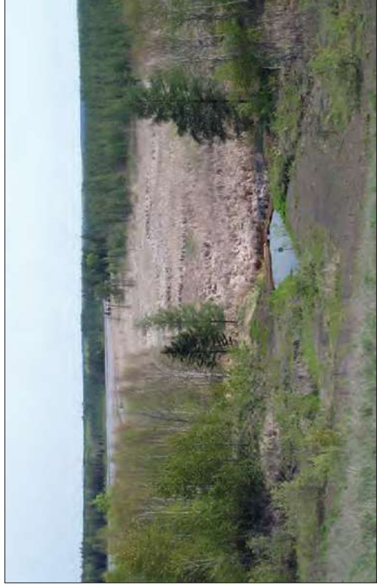
Water seeping out of the Minntac tailings basin and moving toward the Sandy Lakes in Minnesota.
