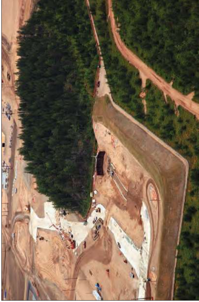
Access portal for the Eagle mine is drilled into the base of Eagle Rock, a sacred site to tribal people. (photo courtesy of Chauncey Moran)
