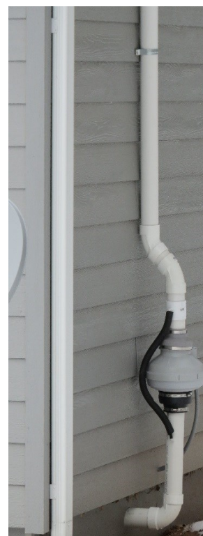
Figure 1: Radon Mitigation Fan used for lowering levels on Housing Authority unit.
